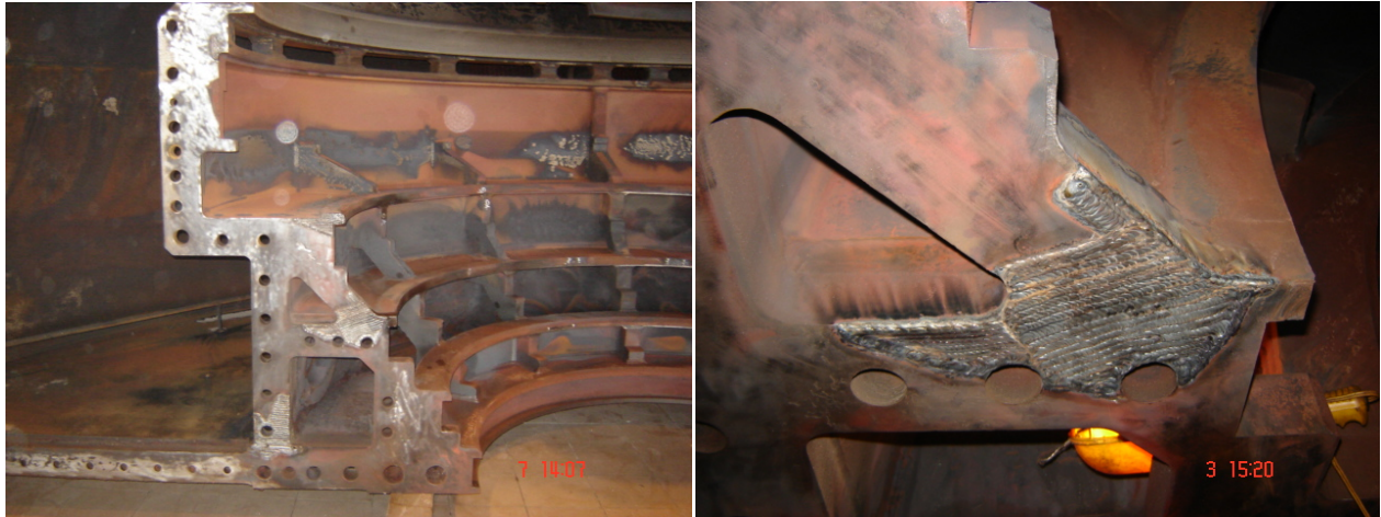
Figure 7 Water Induction Damage and Rubbing Repairing
