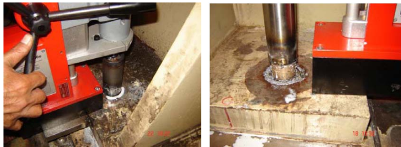
Figure 8 Expanding the anchor-bolt holes of Base plate
