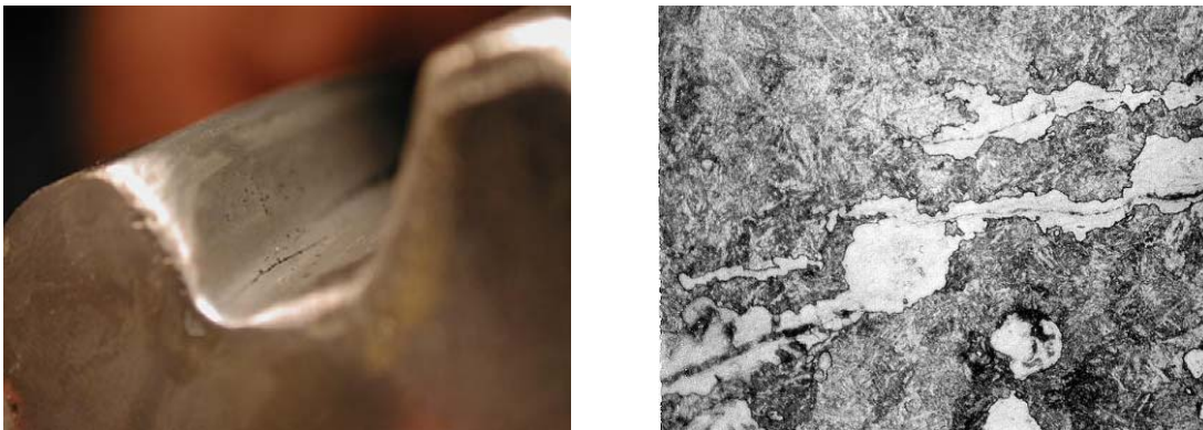
Figure 1 Example of Stress Corrosion Cracking on LP rotor groove
